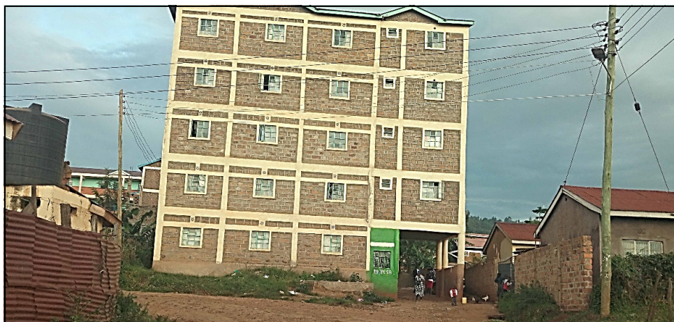
FIGURE II. A BUILDING FLOUTING PHYSICAL PLANNING STANDARDS IN DARAJA MBILI
